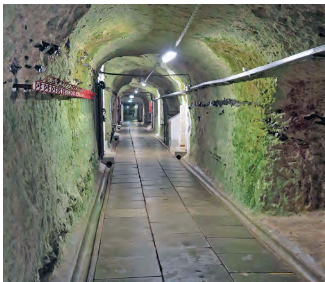
Unlined tunnel within Stevns Fort; cut in chalk, a layer of flints can easily be discerned. The left foreground has coat hooks in situ, middle distance right is the tiled surround of a urinal
